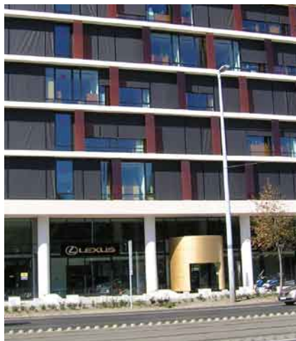
The facade of the "K2" building shown here uses coloured glass panes embedded in Sikasil® SG-20. Produced by Rollatech, the project is a fine example in the use of designer glass to create a finish of distinction.
