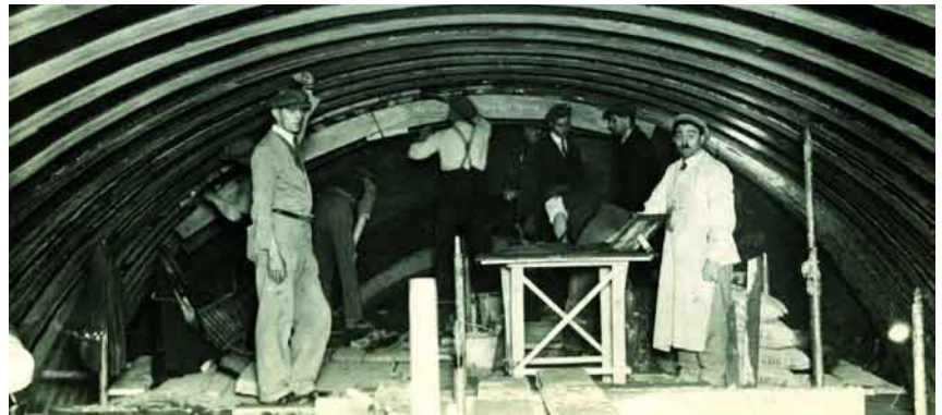
Waterproofing the first Gotthard railway tunnel
