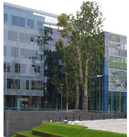
In the Eiffel Office Building (above) Schal Tech created the facade using IG units by Jülichglas
