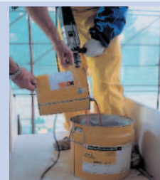
Fig. 6 Transferring the SikaTransfloor®-352 to another container
