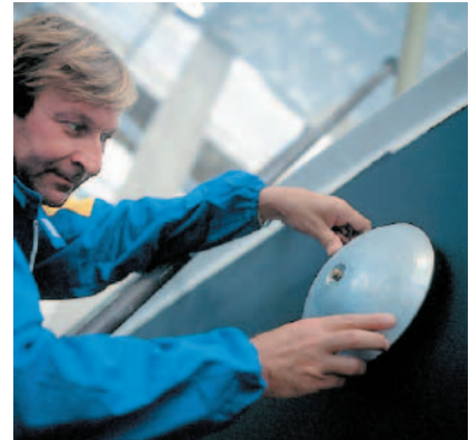
Fig. 2 The anode is fitted
