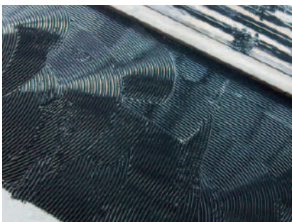
Fig. 12 Sikaflex®-298 applied with a comb spreader
