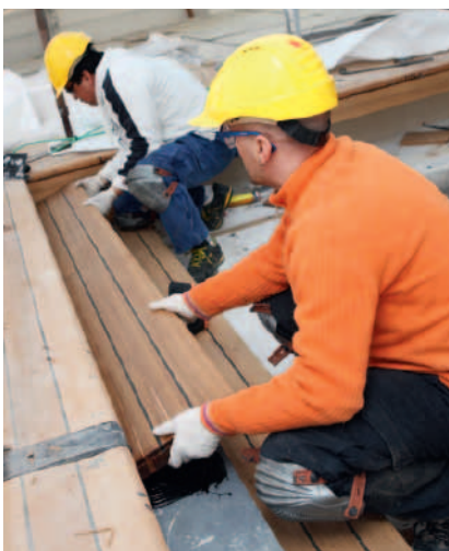
Fig. 13 Putting down the decking
