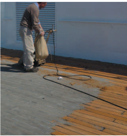
Fig. 20 Sanding the deck
