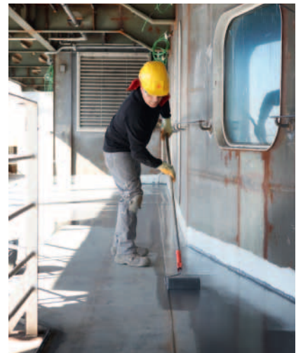
Fig. 3 Applying SikaCor® ZP Primer with a roller
