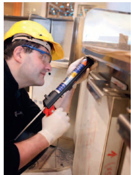
Fig. 4 Application of Sikaflex®-291i
