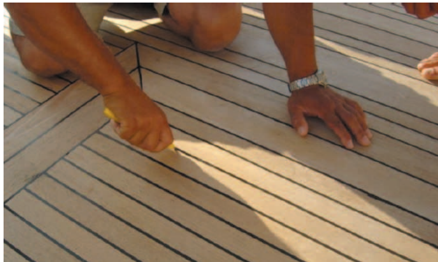
Fig. 34 Using a craft knife to cut along the part of the joint to be removed
