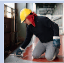
Fig. 8 Spreading the SikaTransfloor®-352
