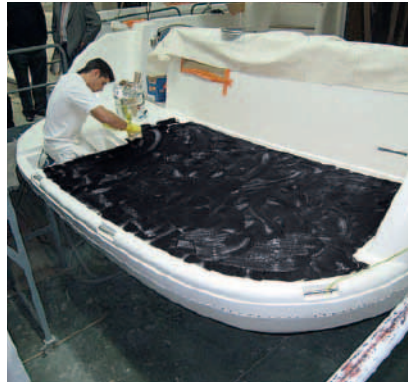
Fig. 25 Application of Sikaflex®-298
