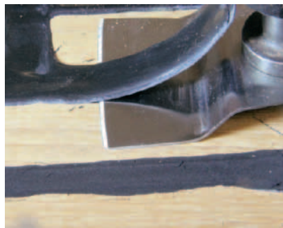
Fig. 49 Picture Removal overstanding Sikaflex®-290i DC with a vibrating scraper power tool
