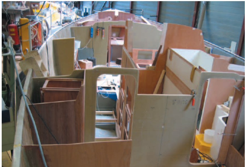
Fig. 2 Lightweight panels being fitted to an open hull
