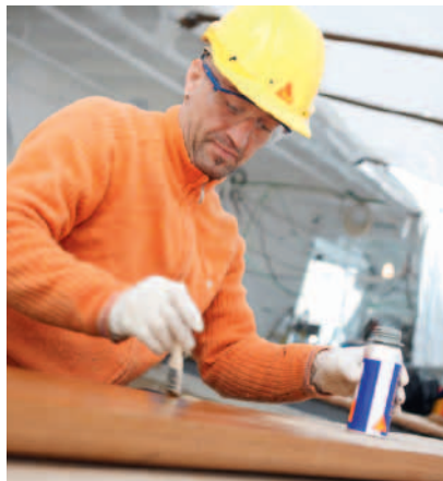
Fig. 10 Carefully applying Sika® MultiPrimer Marine
