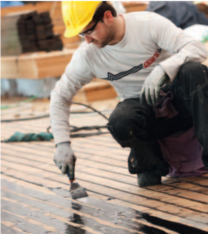
Fig. 19 Compressing Sikaflex®-290i DC with a spatula
