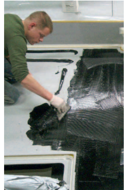
Fig. 55 Application of Sikaflex®-298
