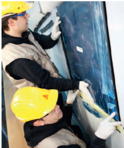
Fig. 3 The window is fitted
