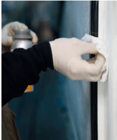
Fig. 1 Cleaning (pre-treatment) of the ceramic ink area with Sika® Aktivator
