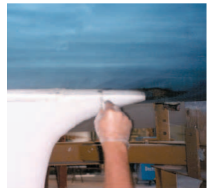
Fig. 3 The joint is tooled off and finished
