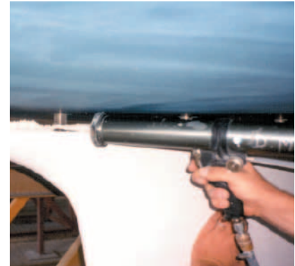
Fig. 2 The adhesive is applied
